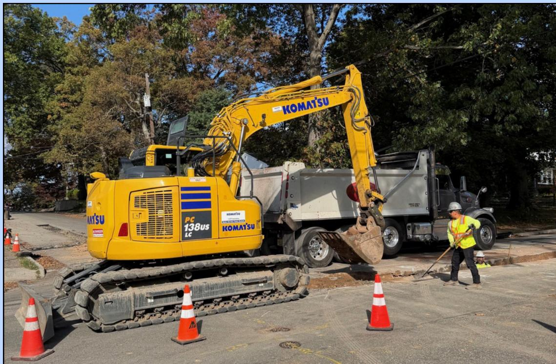
Installing a raw water main that will connect satellite wells to the new PFAS Treatment Facilities.
