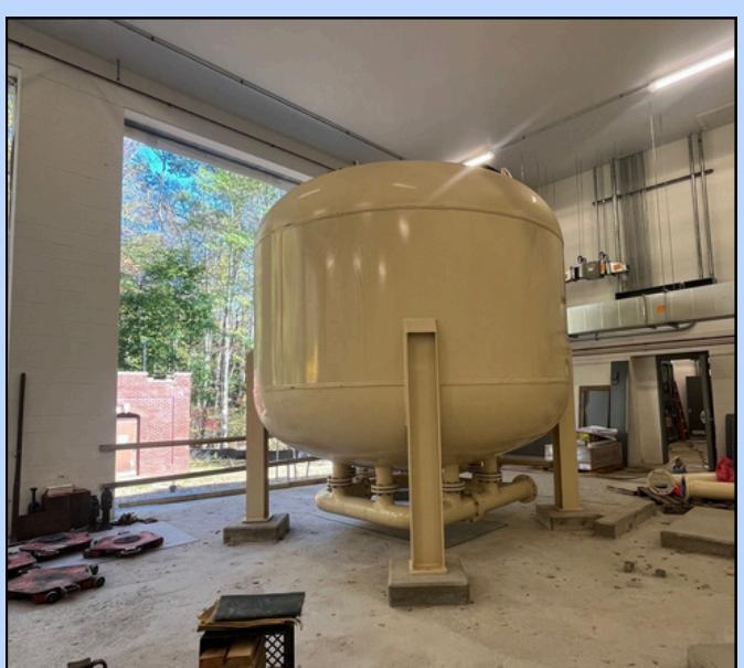
The delivery of granular activated carbon vessels at the Ames PFAS Treatment Facility in Wyckoff.
