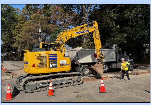
Installing a raw water main that will connect satellite wells to the new PFAS Treatment Facilities.
