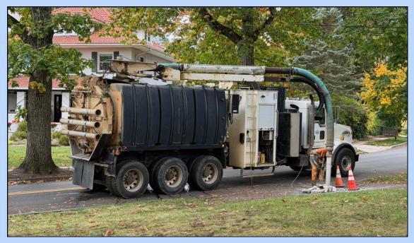
A hydroexcavator identifying the material of a service line that is currently unknown in our records.
