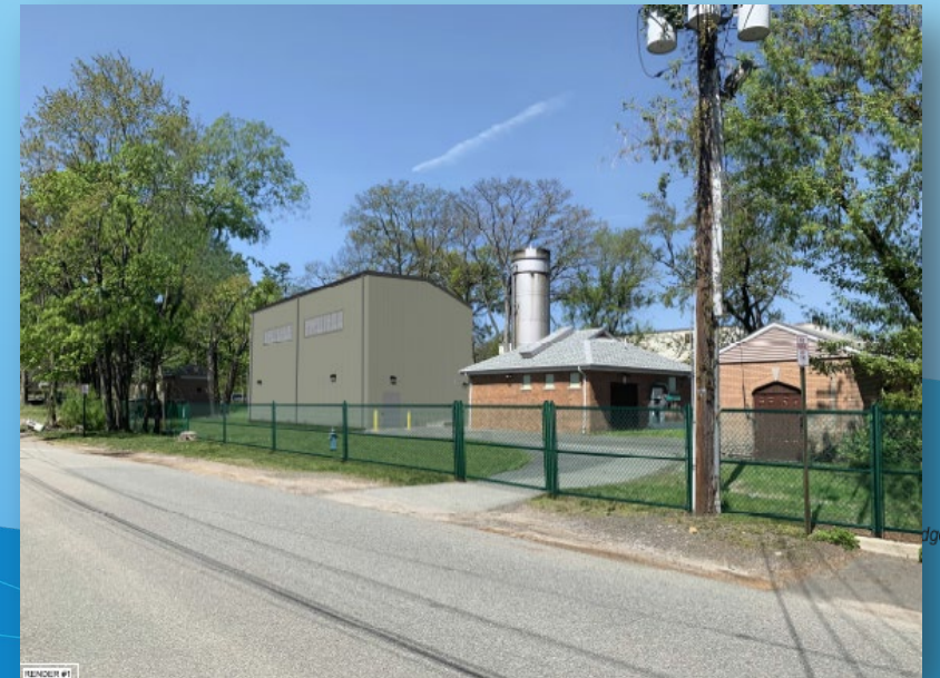
Wortendyke PFAS Treatment Facility
