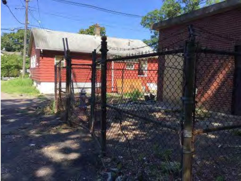
House basement as proposed clear well
