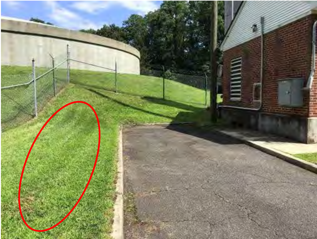
Location of future PVWC interconnect chamber
